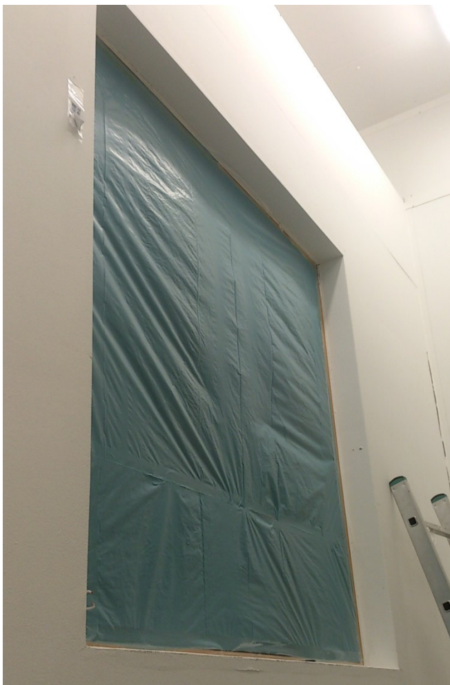
Figure 5-5 Window blinded from the outside by a plastic foil
