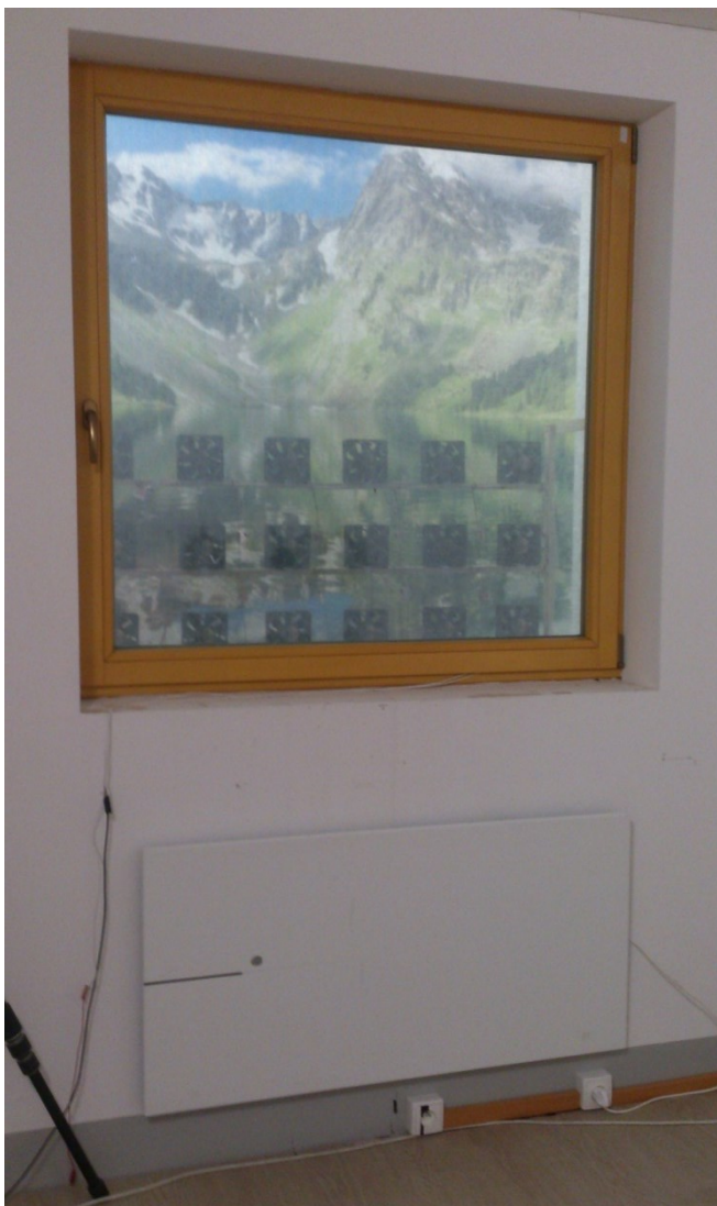
Figure 5-3 View of a window with a window screen from the interior
