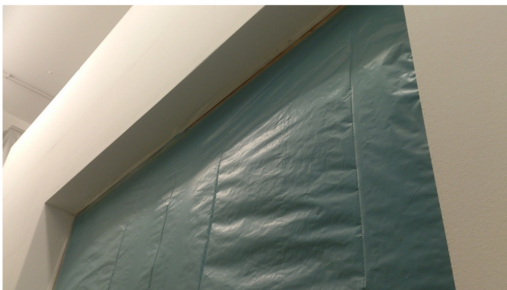
Figure 2-5 Blinds the window with a plastic foil
